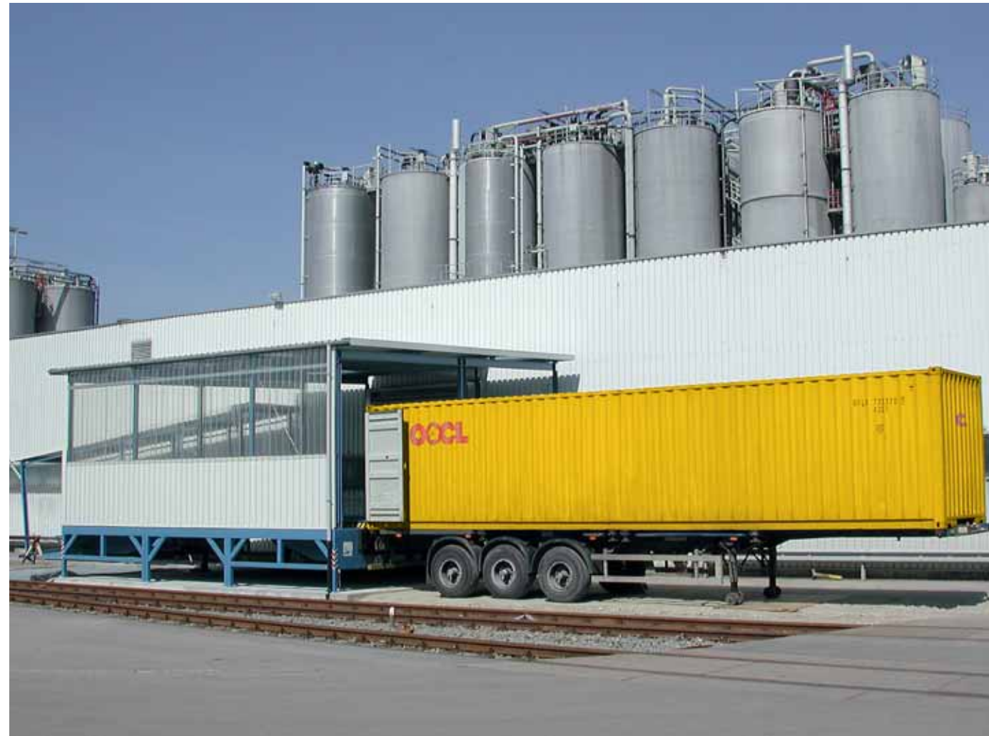
Canopied loading stations with dock levellers and excavation bevel.
